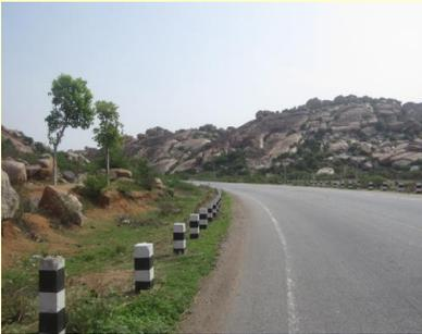
Concrete guide posts are commonly used in Karnataka but they are serious roadside hazards. They should be made highly conspicuous, with reflectors attached to them. When damaged, they should be replaced with white plastic guide posts with large reflective strips on each.
