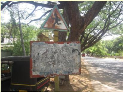
**CLEAR** – the shape and colour of the sign, as well as the legend/symbol, have to be able to be read from a sufficient distance. This warning sign is not clear and should be replaced.
